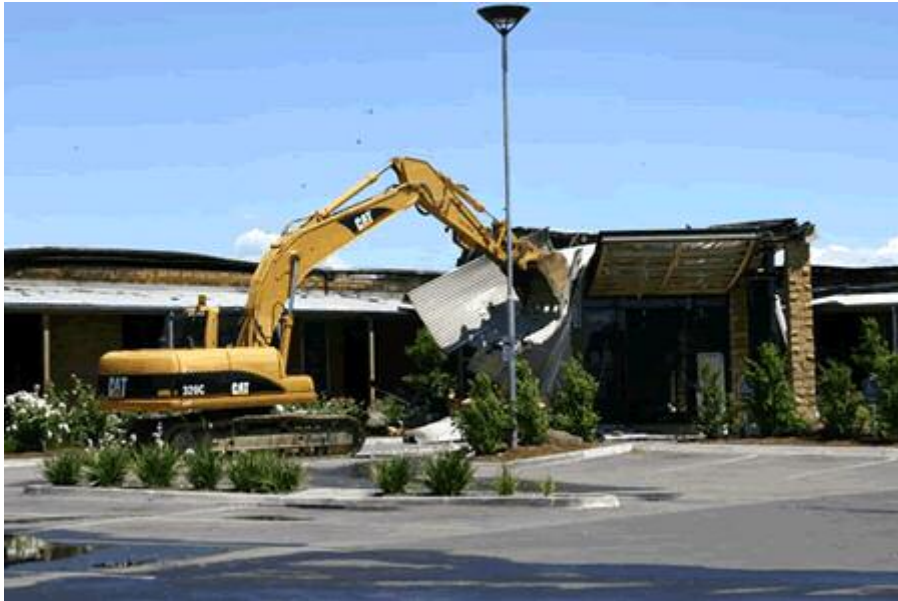
Demolition works continue. Photo: Matt Taranto
